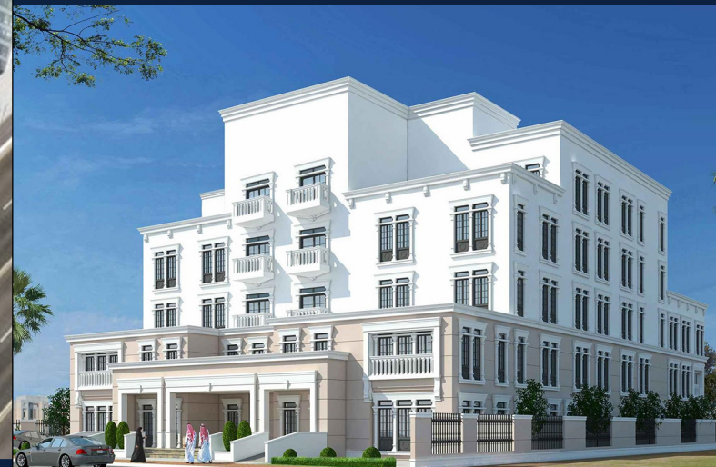
RESIDENTIAL BUILDING A38, LUSAIL
